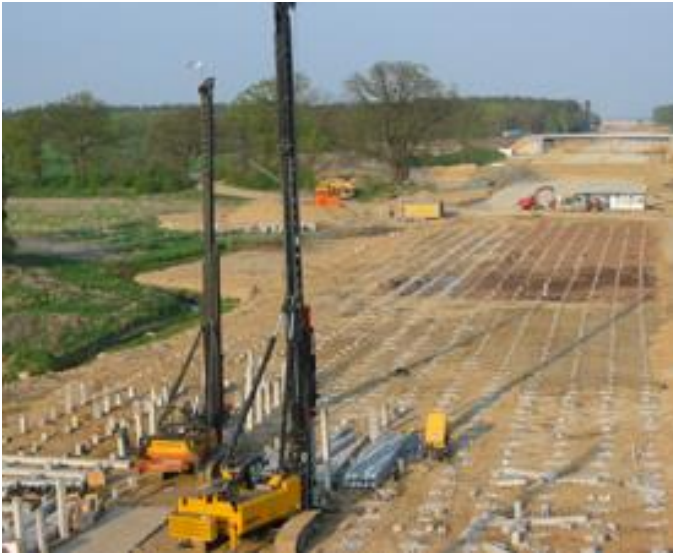
Fig. 5. Building site (Highway A-2).
