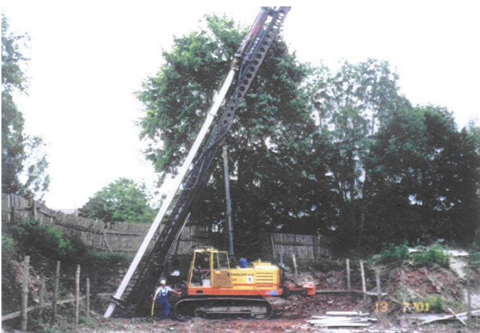
Fig. 7. Driving in of the 15-meter long pile, inclined by 27 deg.
