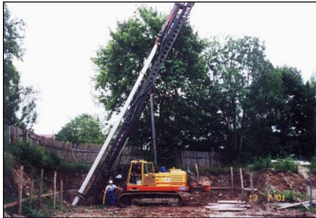
Fig. 2. Driving in of the 15-meter long pile, inclined by 27 deg.
