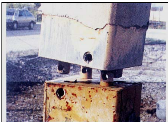
Fig. 3. Steel joints used to join the piles with 40×40cm section.
