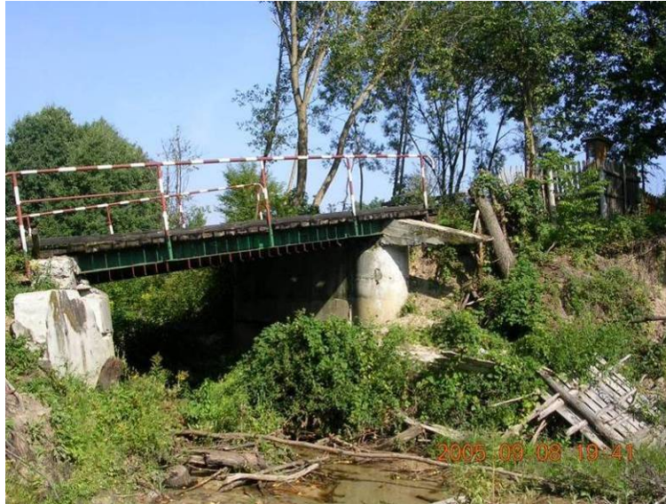
Fig. 1. An overview of the bridge before the reconstruction
