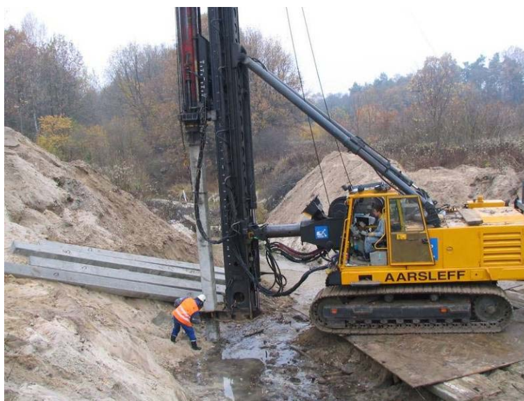
Fig. 4. Driving of 30x30x700cm prefabricated piles
