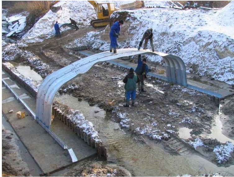
Fig. 5. Steel structure assembling
