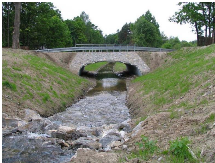
Fig. 7. Bridge overview after the reconstruction
